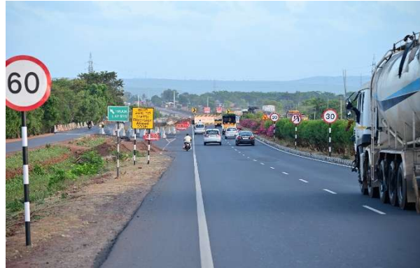
Road Diversion in Day Time
